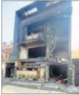
The charred building in Pratap Vihar, Sector II. HT PHOTO
